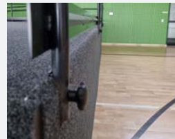
Fascia with Hand Rail cut away
