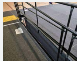
Access Ramp at rear of Stage
