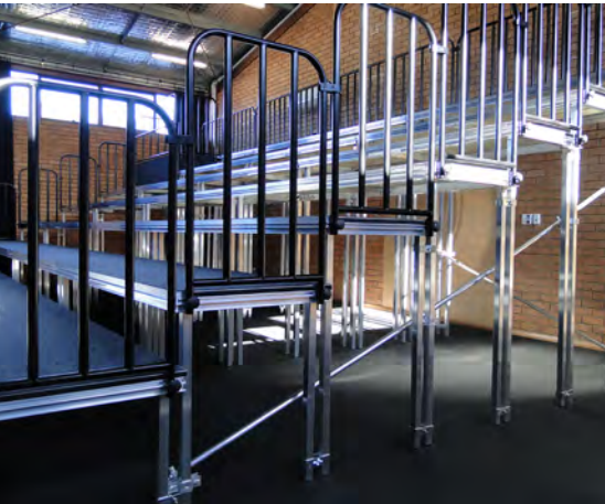
Sway Bracing with Sway Brace Clamps
